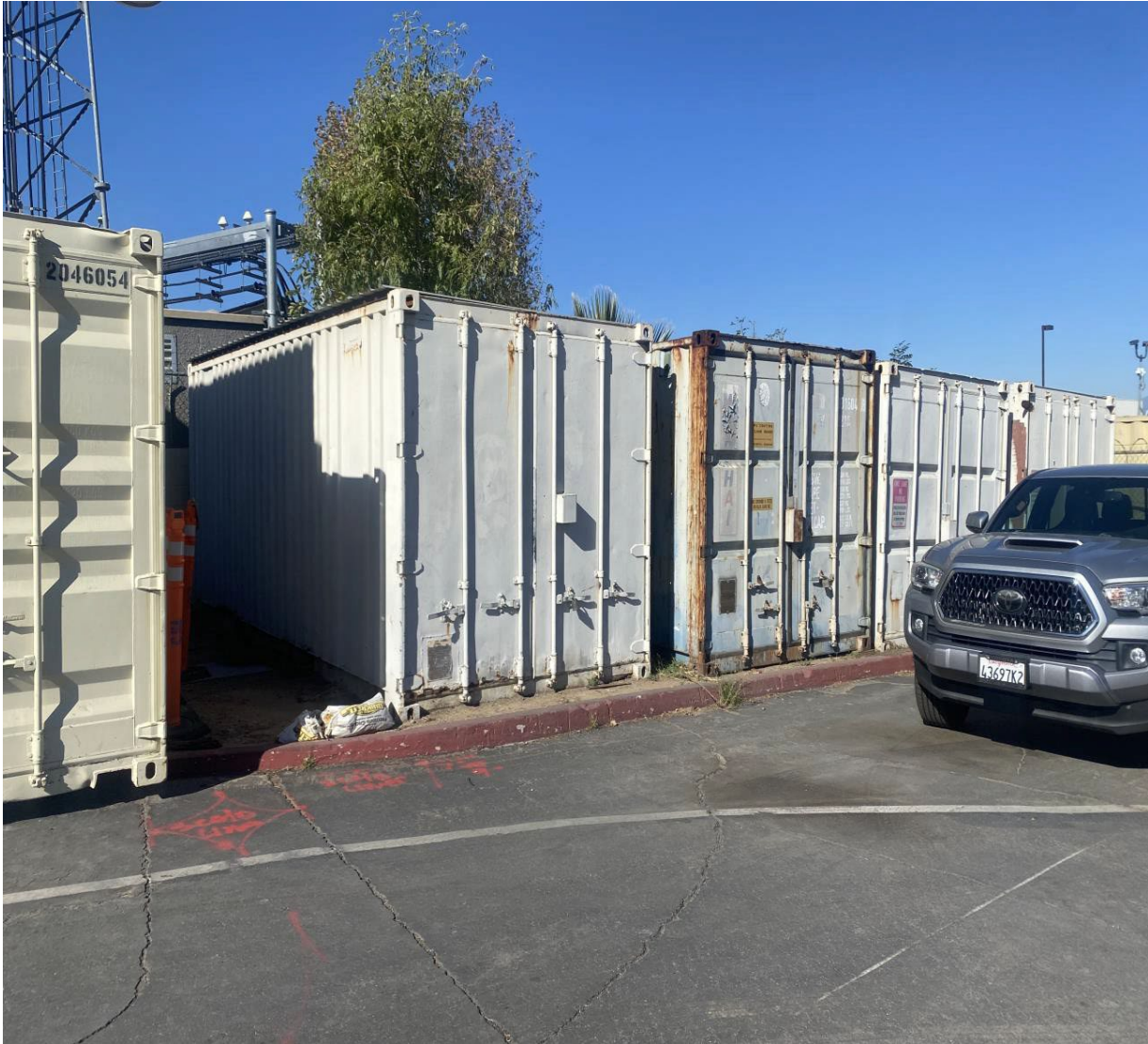
Figure 5: Photo showing curb that needs to be removed and the dirt area where asphalt needs to be installed and where the relocatable building will be placed.
